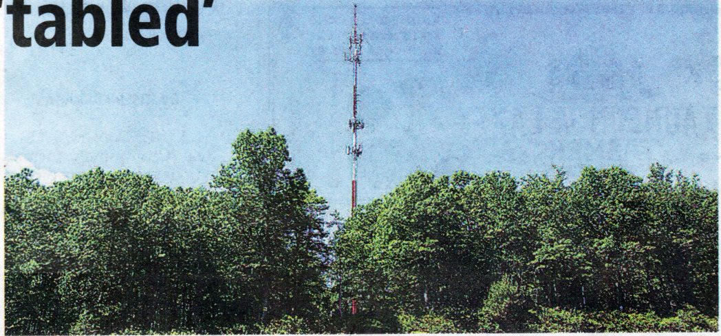
A cell tower, like this one near Wurtsboro, has been in development for months. It was planned to be installed near Rock Hill but it has now been postponed.
